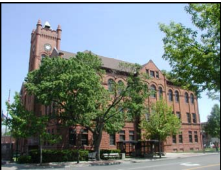
1. / The Champaign County Courthouse , at 101 East Main Street, was built in 1901. This Joseph Royer design, with brick and sandstone exterior is the fifth Champaign courthouse.
