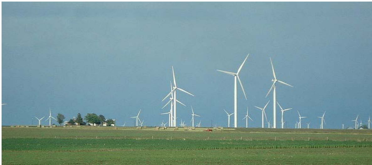
1.65 MW/269 foot rotor diameter/214 foot system height
