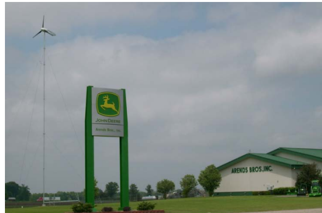
5.0 kW/21 foot rotor diameter/115.5 foot system height
