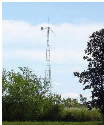
20 kW/100 foot system height
