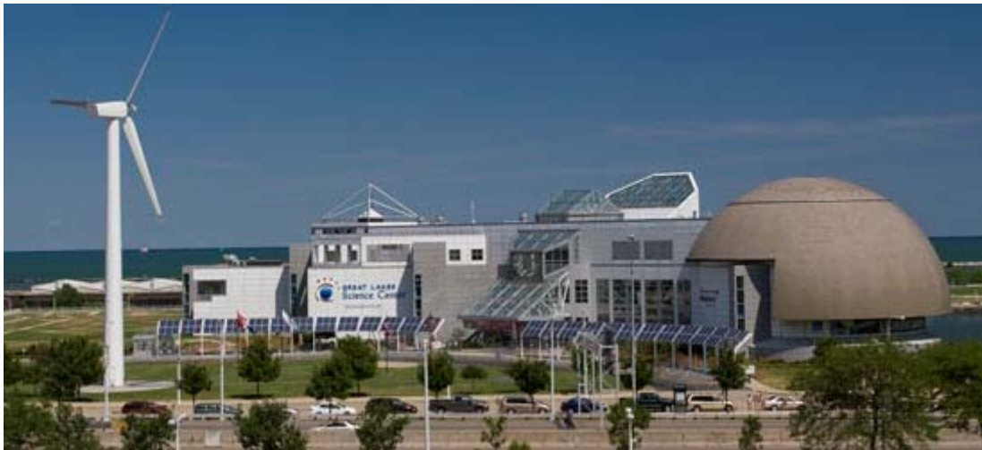
225 kW/88.6 foot rotor diameter/150 foot system height
