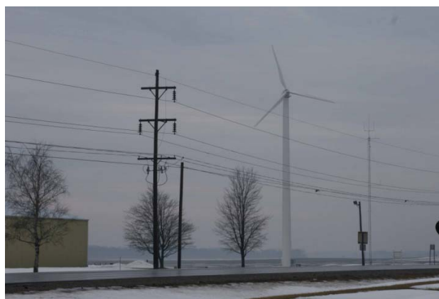
100 kW/70 foot rotor diameter/159 foot system height
