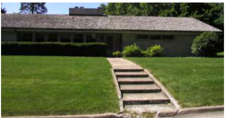
▲ Hindsley House, 1 Montclair Street
