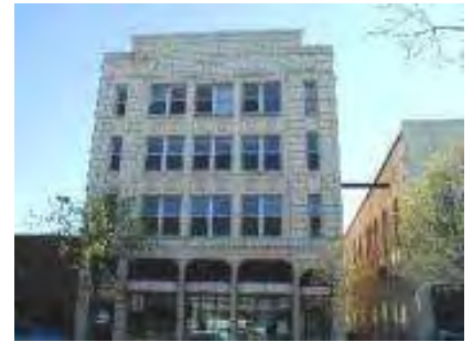
▼ Tiernan's Hall, 115 W. Main Street Built in 1871 with façade designed by Joseph Royer in 1913
