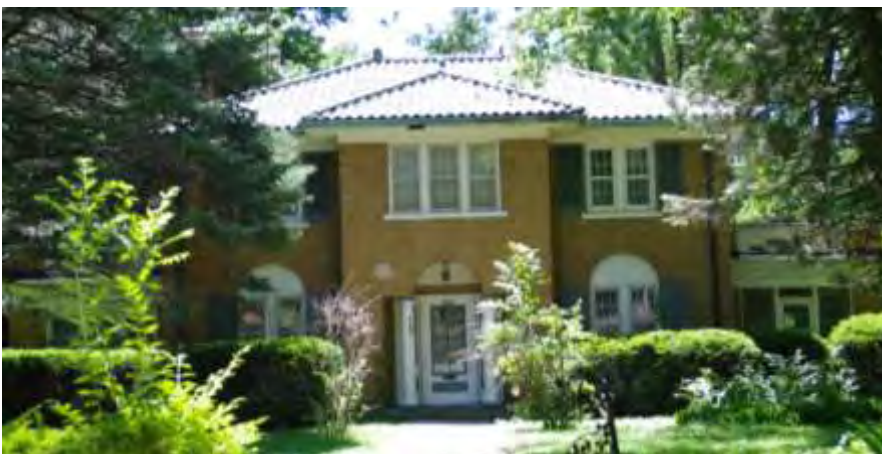
▲ 309 W. Michigan Avenue Built in 1925 in the Mediterranean architectural style
