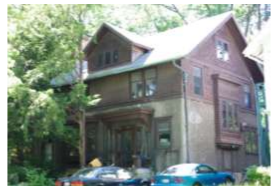
▲ 512 W. Nevada Street Built in 1925 in the Georgian Revival architectural style. The garage of this house has the original garage doors.
