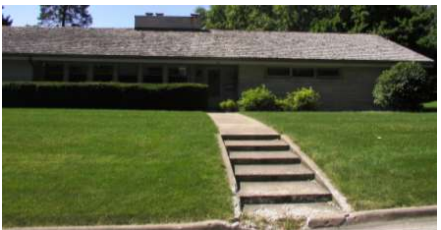
▲ Hindsley House, 1 Montclair Street
