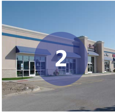
Gateway Shoppes New Construction
