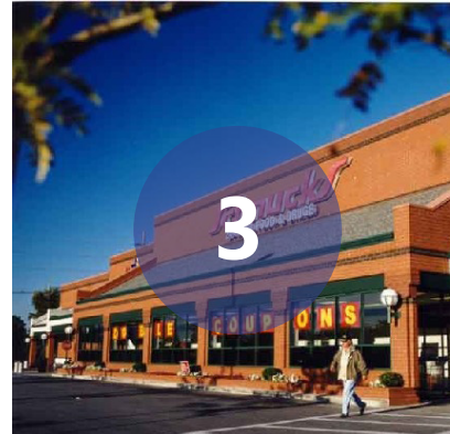
Urbana Crossing / Schnucks Market New Construction
