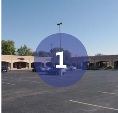
Five Points Commerce Center New Construction
