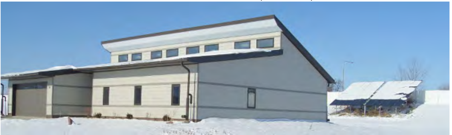
View from Street in winter with solar panels in the rear.
