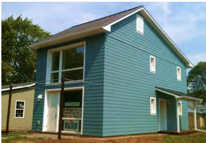
View from the South-East
