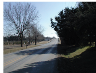
High Cross Road north of I-74 bridge
