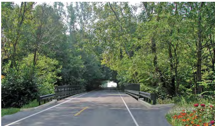
Figure 4-9: Future View 1: Saline Ditch Bridge
