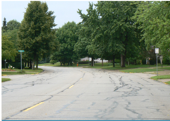
Figure 125 Vine Street north of Windsor Road
