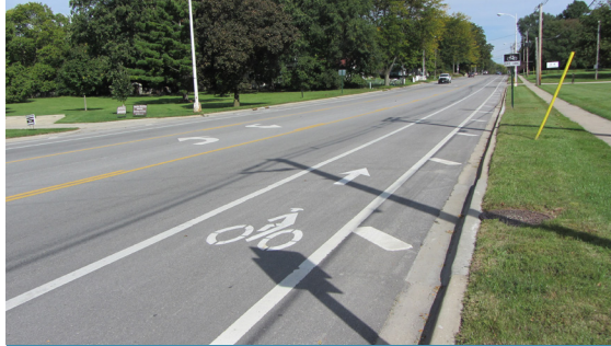
Figure 123 Main Street east of Art Bartell Road
