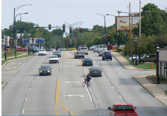
Figure 129 Vine Street south of the Railroad bridge, approaching Main Street
