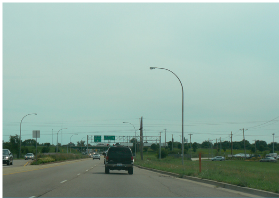
Figure 131 Cunningham Avenue south of O'Brien Drive, approaching I-74
