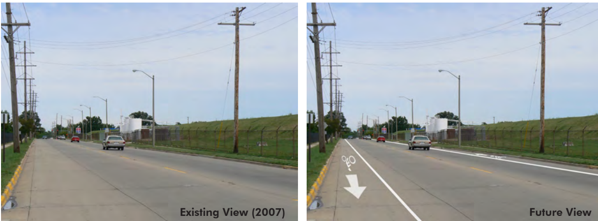
Figure 149 Bradley Avenue east of Goodwin Avenue
