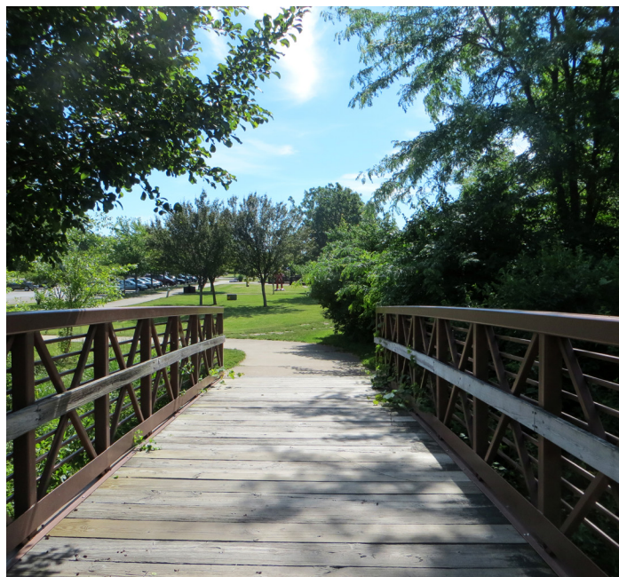
Figure 77 A shared-use path bridge over McCullough Creek in Meadowbrook Park
