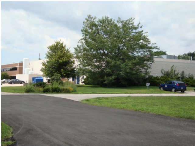
Property north of subject parcel, zoned Industrial.
