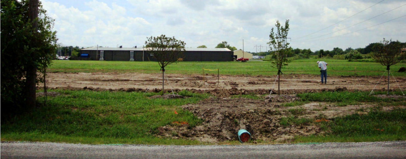
Subject parcel in foreground. Picture taken along Willow Rd., looking West. Photograph shows parking lot construction for building #2.
