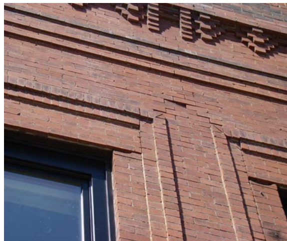
Left & Right: The exterior brick walls at 212 W. Main are exhibit step cracking and deteriorated mortar joints.
