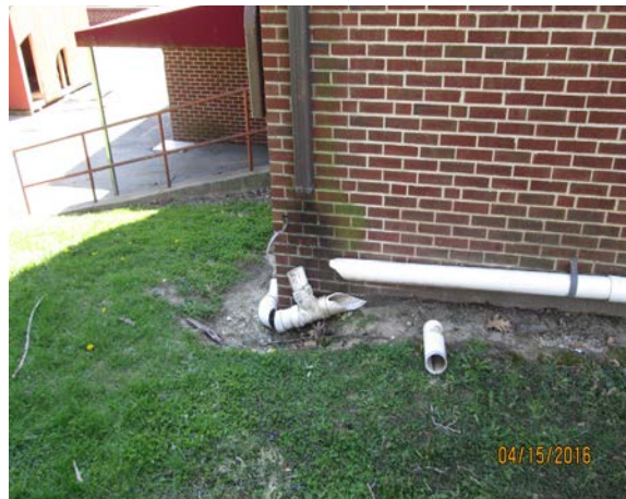
Left & Right: Guttering and downspouts at the vacant Washington School have become dislodged and are broken. (04/15/2016)
