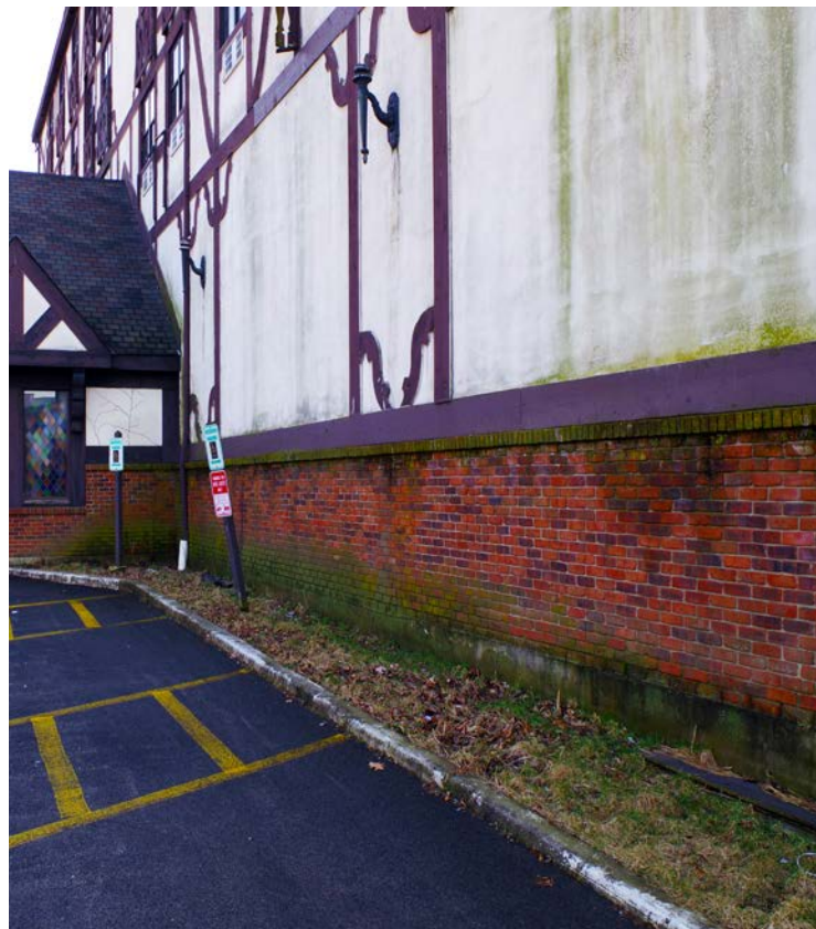
Below: Algae and mold growing on the exterior walls of 201 S. Race. (03/07/2016)
