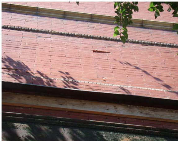
Left: The exterior brick wall at 208 W. Main is in need of tuck-pointing.
