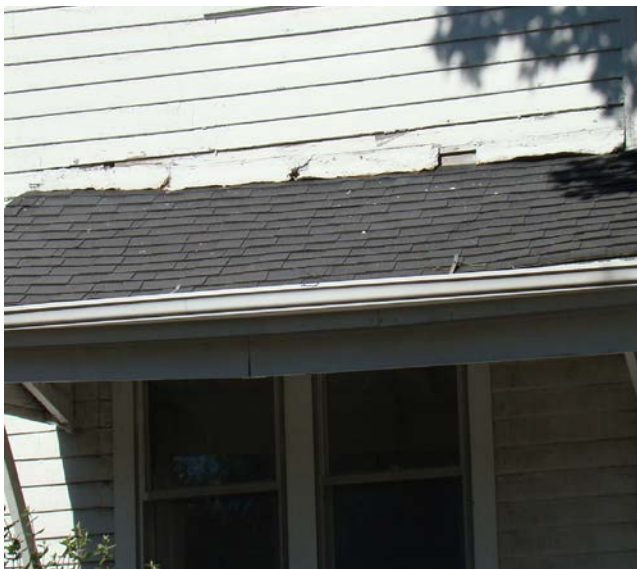
Above: The porch on 206 S. Cedar is sagging and the wood siding has rotted.
