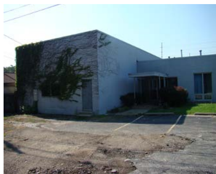
Left: The rear lot for the above property along Vine Street is also deteriorated.
