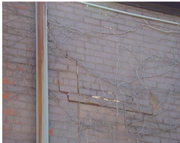
Right: Step cracking in the rear wall at 306 W. Springfield. (03/07/2016)
