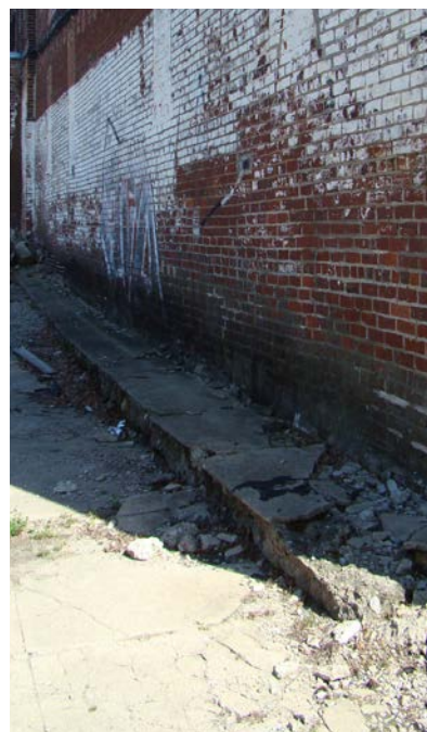
Above and Below: A deteriorated sidewalk located at 119 W. Water Street.
