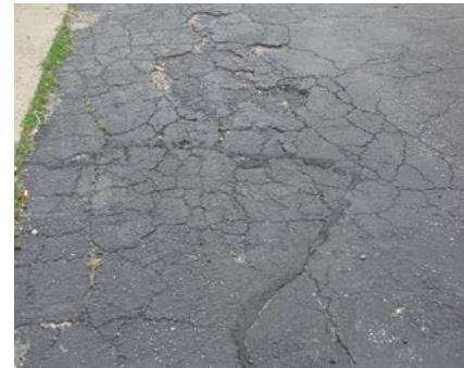
Above: Deteriorated asphalt at 508 S. Vine Street.
