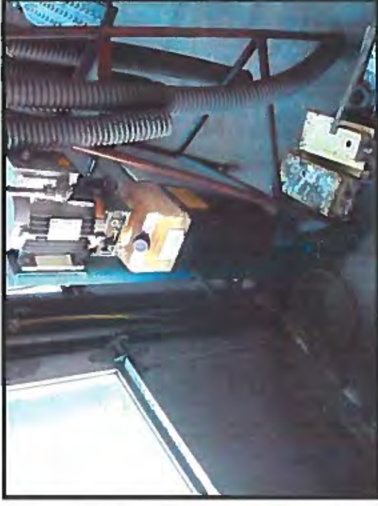
Photo 34: Motor and fluid for underground hydraulic lift
