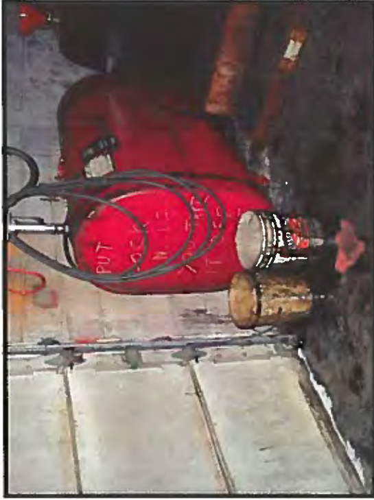
Photo 25: Oil ASTs and stained pavement near exterior wall and overhead door (Photo 8)
