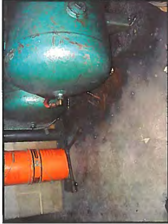
Photo 23: Oil stained pavement and floor drain underneath air compressors (Photo 9)
