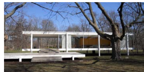
Farnsworth House, Plano, Illinois by architect Mies van der Rohe
